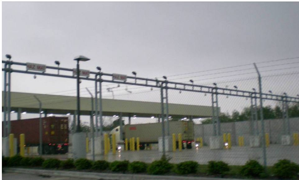
Figure 5. View of truck lanes at the new entry pre-check facility.
